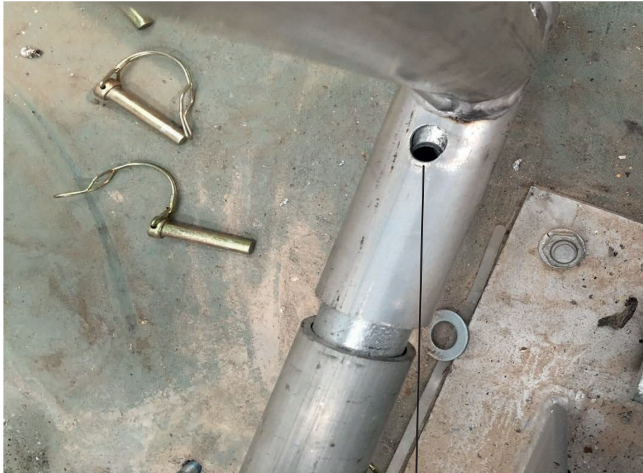
Lower chord aluminium tube elongation post load evident
