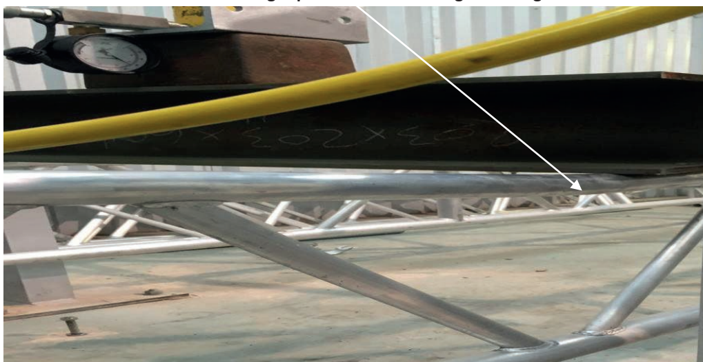
3.6.1 Showing top chord failure through crushing
